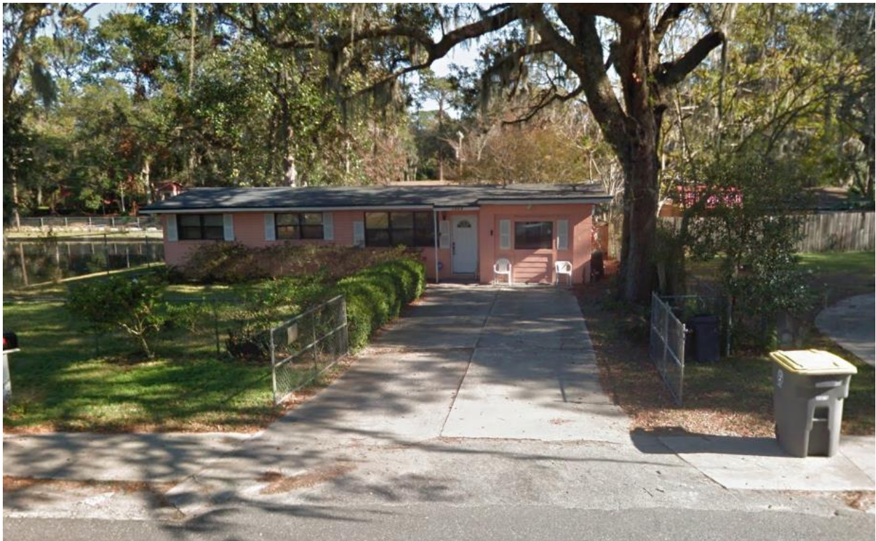
Adjoining property to the east across Foster Drive
